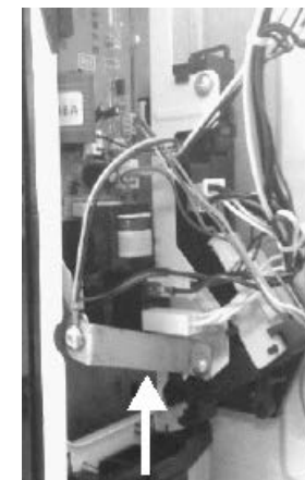
Bracket (and ground wire) secured
