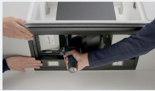
Alternatively, the hood can also be installed in a furniture cutout from below, for example, if a light panel is mounted below the cabinet. In this case, installation requires a second person.
