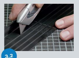
Cut the lower filler strips according to the cupboard depth and mount those accordingly.
